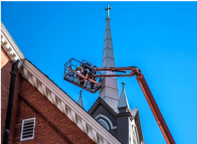
Power-Chiseling the fogged plexiglass panels from the nine windows in the front of the church. To be replaced with clear Lexan panels
