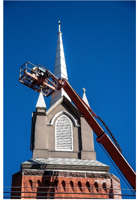
Securing the Aluminum plates encasing the spire. Some have been replaced.
