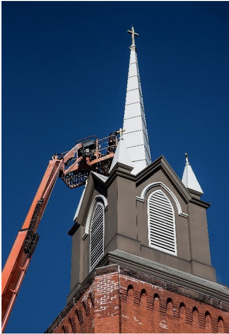
Securing the Aluminum plates encasing the spire. Some have been replaced.
